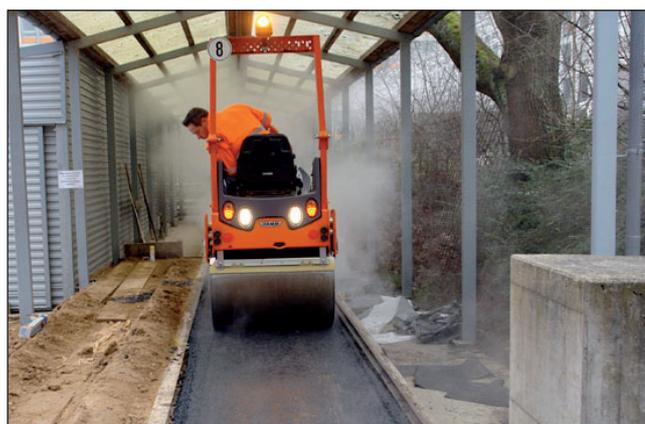
Fig. 4.: Asphalt installation and compaction
